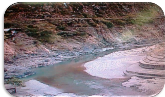
Fig. 1 c TR 3. Regulated stretch 20 km d/s of Koti Dam (close to Chhivrau PH)
